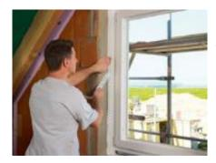
The white coloured, single-sided high-performance adhesive tape Fentrim 20 is the optimal solution for permanent airtight bonding of window and door frames in **solid construction from the inside**.
